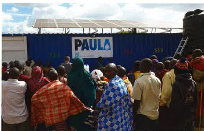
Residents of the village in front of the PAULA drinking water system, on whose roof the solar panels are installed
